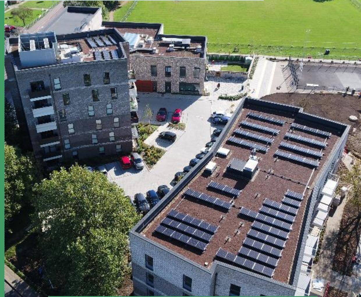
Alumasc Roofing – Hydrotech & Blackdown Green Roofs Buchan Street and The Meadows Community Centre, Cambridge
